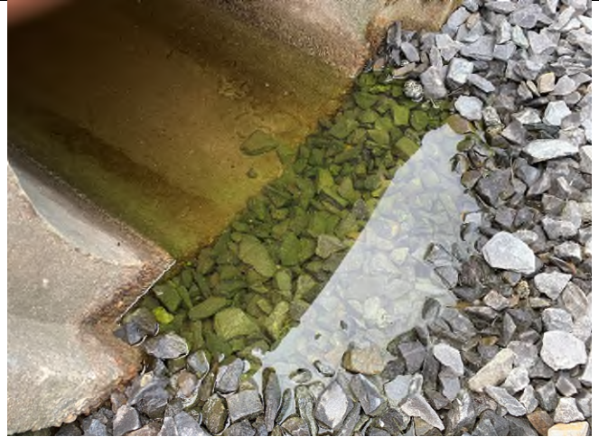
29 Gundalow -1 (Drainage Area)
