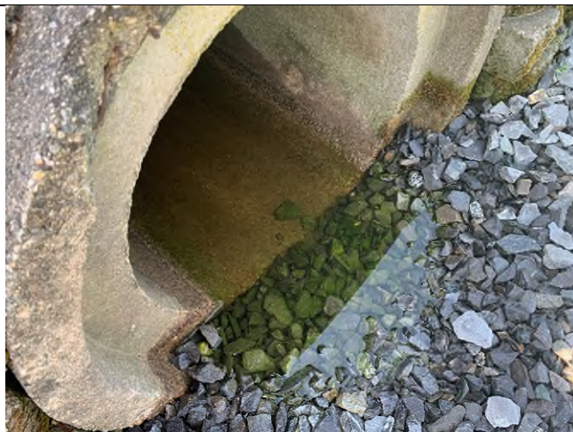
29 Gundalow -1 (Drainage Area)
