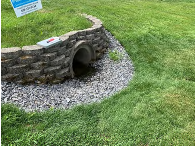
29 Gundalow -1 (Drainage Area)
