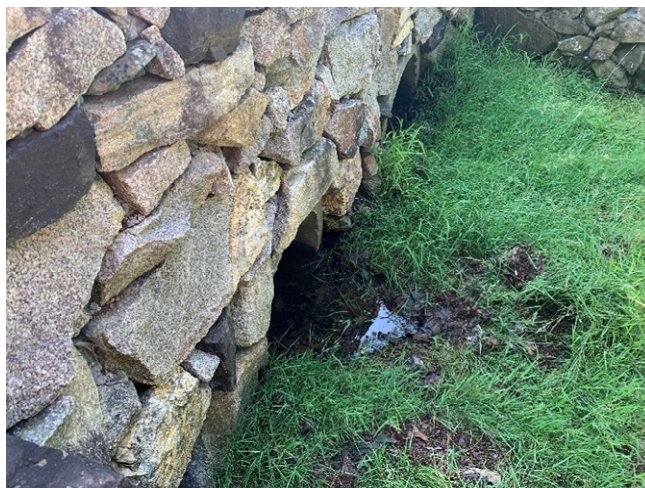
4 Brickyard Circle - 1 (Drainage Course)
