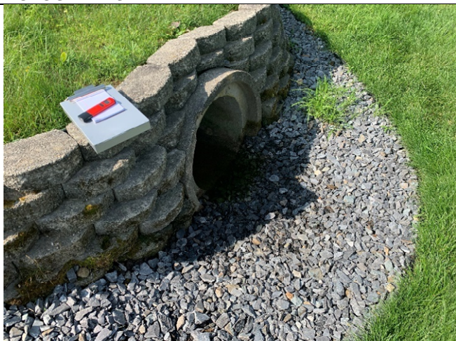
29 Gundalow -1 (Drainage Area)
